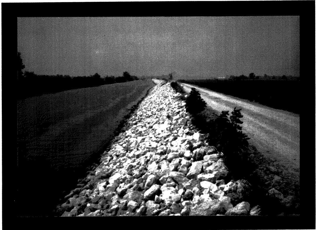
Wards Canal - Rehabilitated levee.
