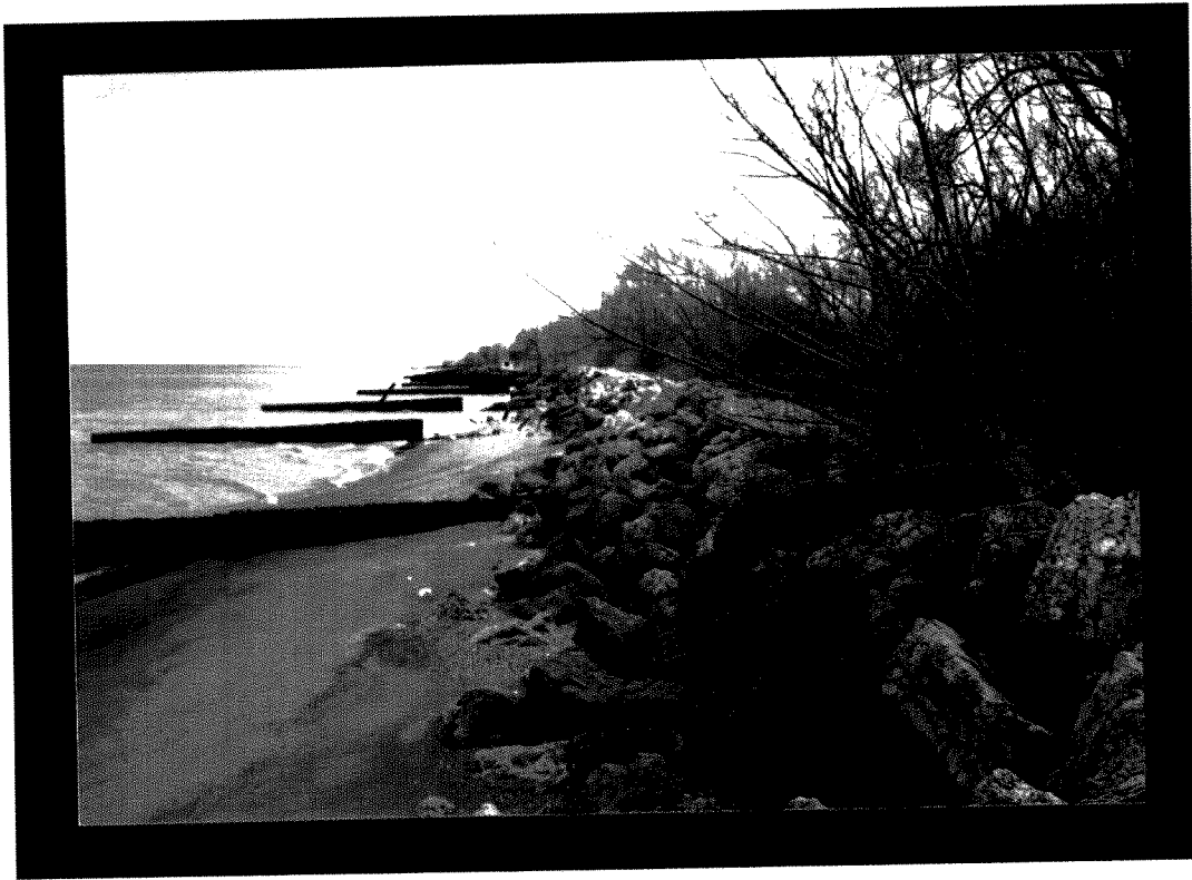
Approximately at sta. 63+00, facing east.
