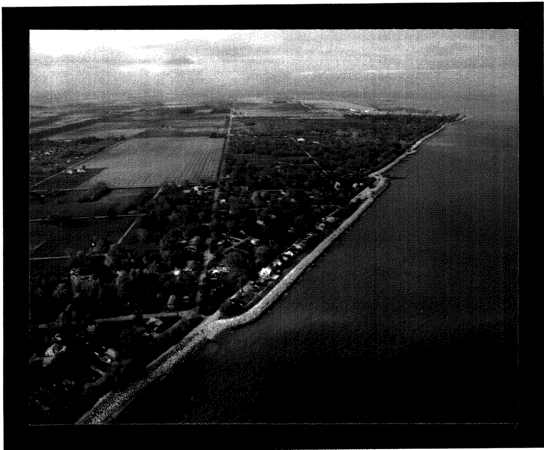
Aerial view of approximately sta. 58+50 to end of project.
