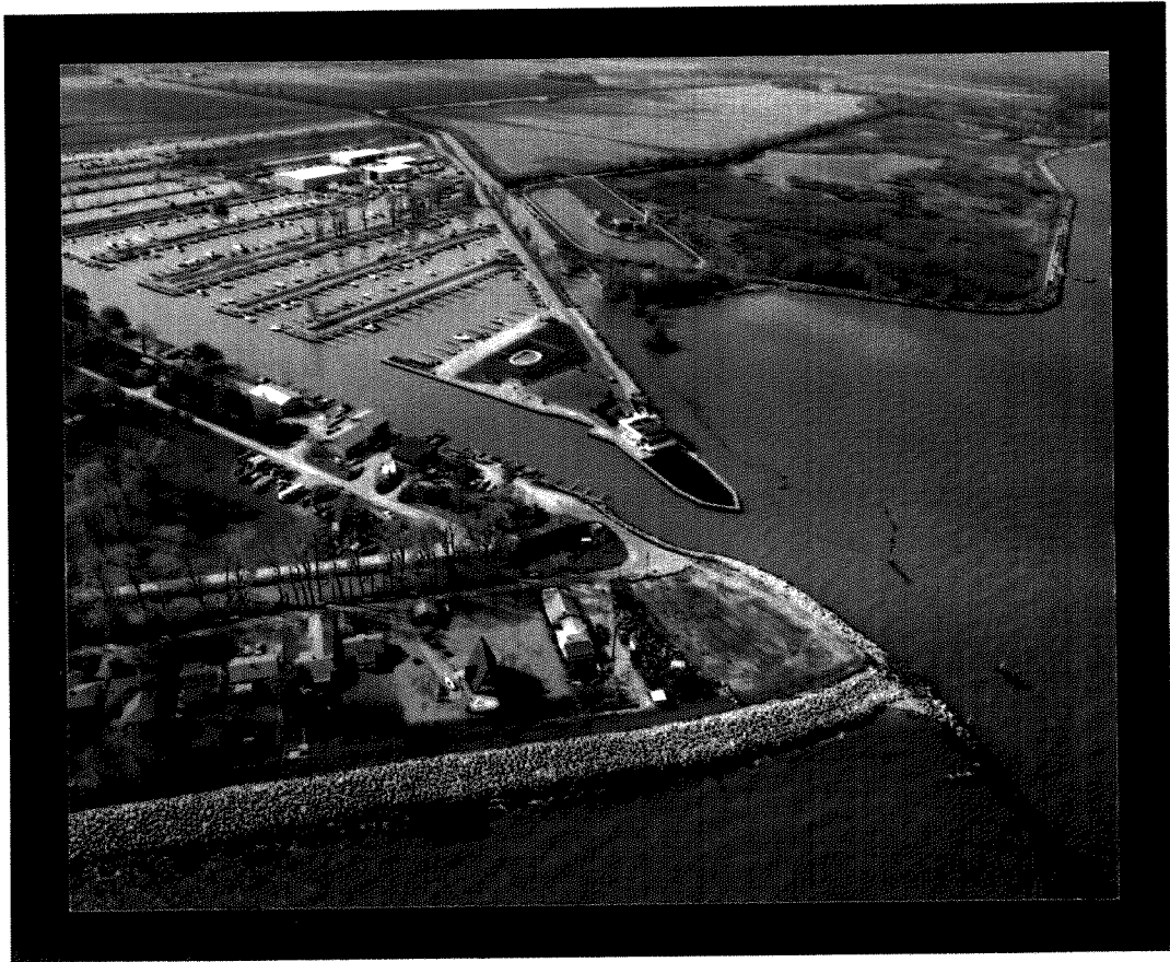
Cooley Canal - Aerial view of end of project.
