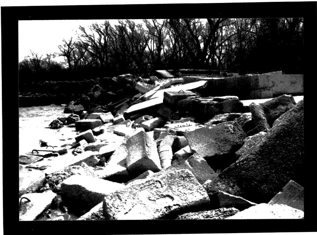
Approximately at sta. 97+00, facing east.
