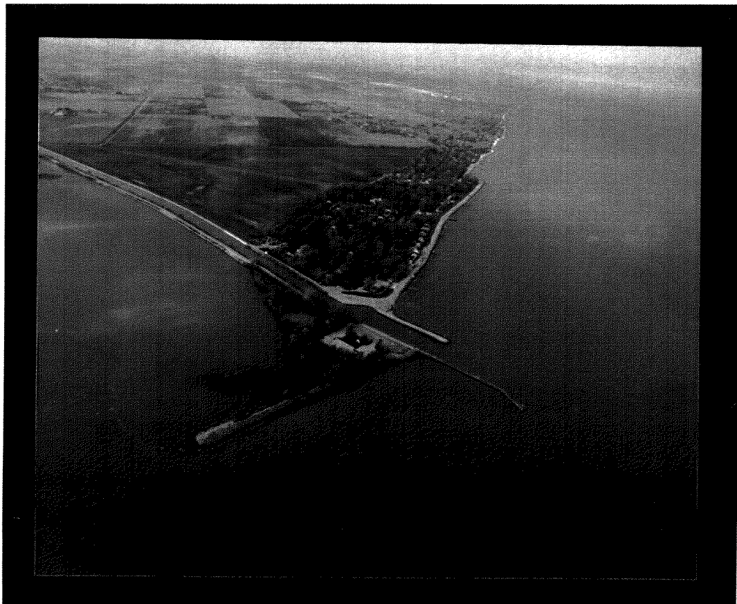
Aerial view of Wards Canal and rest of project.
