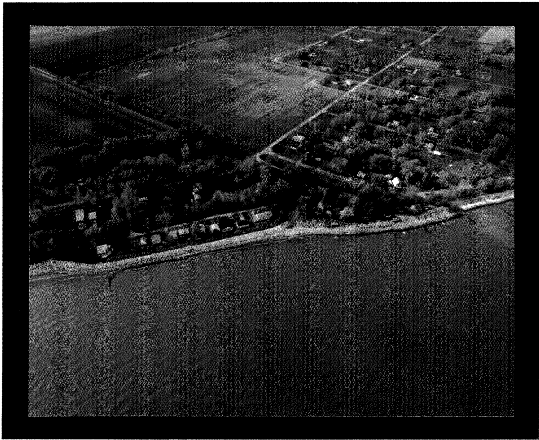
Aerial view of sta. 37+50 to sta 51+50, approximately.
