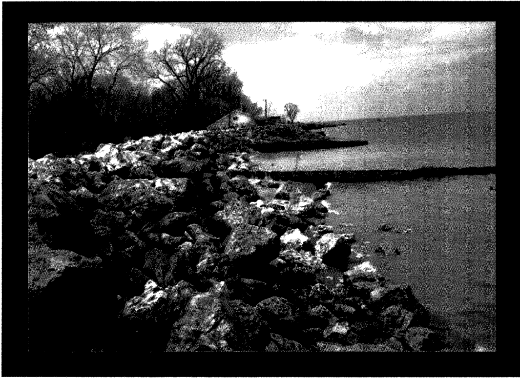
Approximately at sta. 1+08, facing west.
