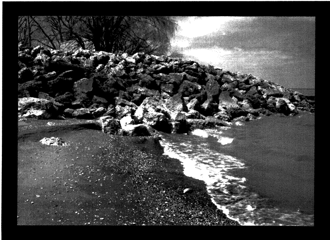
Approximately at sta. 63+00, facing west.
