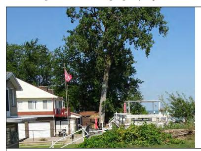
Inspect ID: OH29\_2020\_r\_0019 Title: USACE\_CELRB\_OH29\_2020\_r\_0019\_1.jpg Rated Item: 12. Riprap Revetments & Bank Protection Caption: Rating: Unacceptable; Remarks: Trees and woody vegetation on levee crown and levee landside slope between 12727 and 12743 Lagoon Drive.; Action: Remove trees and woody vegetation from riprap. Perform regular maintenance to prevent further unwanted vegetation development.; Station\_1: 1+73
