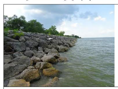
Inspect ID: OH29\_2020\_r\_0027 Title: USACE\_CELRB\_OH29\_2020\_r\_0027\_1.jpg Rated Item: 12. Riprap Revetments & Bank Protection Caption: Rating: Acceptable; Remarks: Riprap on levee waterside slope along Corduroy Road is in acceptable condition.; Action: NA; Station\_1: 52+53
