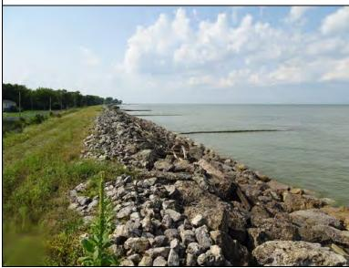
Inspect ID: OH29\_2020\_r\_0034 Title: USACE\_CELRB\_OH29\_2020\_r\_0034\_1.jpg Rated Item: 12. Riprap Revetments & Bank Protection Caption: Rating: Acceptable; Remarks: Riprap on levee waterside slope is in acceptable condition along Lakeway Drive beween Rialto Drive and Park Colony Boulevard.; Action: NA; Station\_1: 96+73; Station\_2: 100+00
