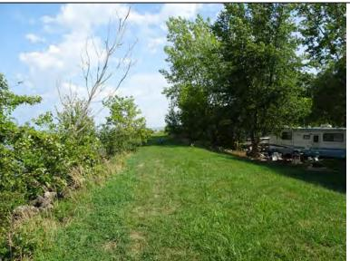
Inspect ID: OH29\_2020\_r\_0036 Title: USACE\_CELRB\_OH29\_2020\_r\_0036\_2.jpg Rated Item: 1. Unwanted Vegetation Growth Caption: Rating: Unacceptable; Remarks: Trees and woody vegetation on both levee side slopes at 11227 Dyke Road.; Action: Remove trees and woody vegetation; establish proper sod cover.; Station\_1: 130+53; Station\_2: 127+10
