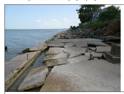
Inspect ID: OH29\_2020\_r\_0024 Title: USACE\_CELRB\_OH29\_2020\_r\_0024\_1.jpg Rated Item: 12. Riprap Revetments & Bank Protection Caption: Rating: Unacceptable; Remarks: Riprap has been removed from levee waterside slope over the distance of approx. 120' near concrete slab, just west of 12153 Corduroy Road.; Action: Replace borken up concrete slab with proper riprap. Should be placed from waterside toe to top of crest.; Station\_1: 50+60
