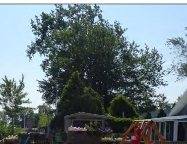
Inspect ID: OH29\_2020\_r\_0019 Title: USACE\_CELRB\_OH29\_2020\_r\_0019\_2.jpg Rated Item: 12. Riprap Revetments & Bank Protection Caption: Rating: Unacceptable; Remarks: Trees and woody vegetation on levee crown and levee landside slope between 12727 and 12743 Lagoon Drive.; Action: Remove trees and woody vegetation from riprap. Perform regular maintenance to prevent further unwanted vegetation development.; Station\_1: 1+73
