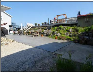
**Inspect ID:** OH29\_2020\_r\_0020 **Title:** USACE\_CELRB\_OH29\_2020\_r\_0020\_1.jpg **Rated Item:** 3. Encroachments **Caption:** Rating: Unacceptable; Remarks: Unauthorized alteration: multiple decks and stairs along both levee side slopes and crown from 12659 to 12743 Lagoon Drive. Riprap has been removed or displaced for decks and stairs. Proper operations and maintenance is impeded.; Action: Remove or Submit Section 408 Alteration Request to USACE.; Station\_1: 0+10; Station\_2: 5+07
