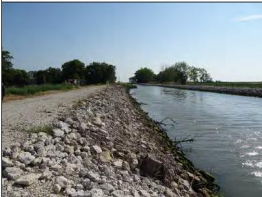
**Inspect ID:** OH29\_2020\_r\_0002 **Title:** USACE\_CELRB\_OH29\_2020\_r\_0002\_2.jpg **Rated Item:** 12. Riprap Revetments & Bank Protection **Caption:** Rating: Acceptable; Remarks: Riprap on levee waterside slope from Toulon Drive to project limit.; Action: NA; Station\_1: -47+80; Station\_2: -11+00
