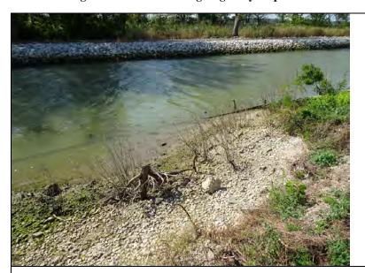
**Inspect ID:** OH29\_2020\_r\_0008 **Title:** USACE\_CELRB\_OH29\_2020\_r\_0008\_1.jpg **Rated Item:** 13. Revetments other than Riprap **Caption:** Rating: Unacceptable; Remarks: SSP wall failure at Wards Canal levee waterside toe threatens dike integrity 300' upstream of canal entrance.; Action: Repair and stabilize SSP wall.; Station\_1: -4+00
