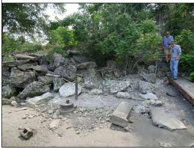
**Inspect ID:** OH29\_2020\_r\_0024 **Title:** USACE\_CELRB\_OH29\_2020\_r\_0024\_2.jpg **Rated Item:** 12. Riprap Revetments & Bank Protection **Caption:** Rating: Unacceptable; Remarks: Riprap has been removed from levee waterside slope over the distance of approx. 120' near concrete slab, just west of 12153 Corduroy Road.; Action: Replace borken up concrete slab with proper riprap. Should be placed from waterside toe to top of crest.; Station\_1: 50+60
