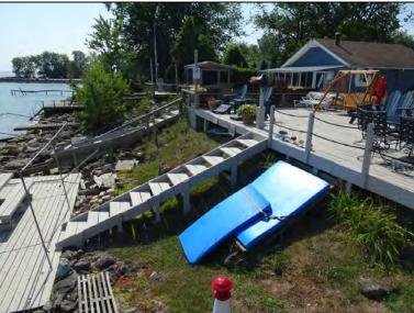
**Inspect ID:** OH29\_2020\_r\_0020 **Title:** USACE\_CELRB\_OH29\_2020\_r\_0020\_3.jpg **Rated Item:** 3. Encroachments **Caption:** Rating: Unacceptable; Remarks: Unauthorized alteration: multiple decks and stairs along both levee side slopes and crown from 12659 to 12743 Lagoon Drive. Riprap has been removed or displaced for decks and stairs. Proper operations and maintenance is impeded.; Action: Remove or Submit Section 408 Alteration Request to USACE.; Station\_1: 0+10; Station\_2: 5+07
