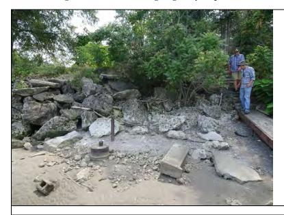
**Inspect ID:** OH29\_2020\_r\_0023 **Title:** USACE\_CELRB\_OH29\_2020\_r\_0023\_1.jpg **Rated Item:** 1. Unwanted Vegetation Growth **Caption:** Rating: Unacceptable; Remarks: Trees and woody vegetation on levee landside slope and crown at concrete slab, just west of 12153 Corduroy Road.; Action: Remove trees and woody vegetation. Perform regular maintenance to prevent further unwanted vegetation development.; Station\_1: 50+60
