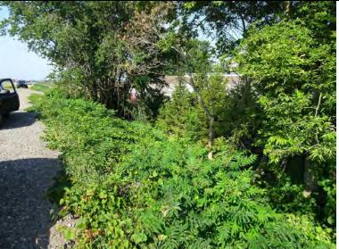
Inspect ID: OH29\_2020\_r\_0010 Title: USACE\_CELRB\_OH29\_2020\_r\_0010\_2.jpg Rated Item: 1. Unwanted Vegetation Growth Caption: Rating: Unacceptable; Remarks: Trees along levee landside slope and toe from Toulon Drive to La Fontaine Drive.; Action: Remove trees from levee slope and toe.; Station\_1: -1+53; Station\_2: -11+00
