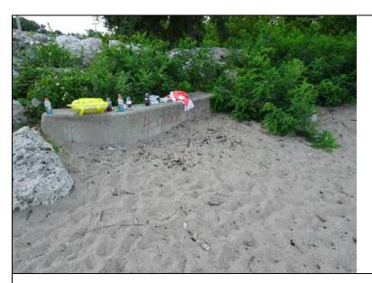
Inspect ID: OH29\_2020\_r\_0029 Title: USACE\_CELRB\_OH29\_2020\_r\_0029\_1.jpg Rated Item: 17. Intake and Discharge Pipelines Caption: Rating: Unacceptable; Remarks: 24" discharge pipe for Dyke Road/Corduroy pump station completely shoaled in. Sponsor digs out sand with shovel. Typically clears out during operation but could be serious issue.; Action: Clear sediments from outfall; consider measures to keep outfall clear of sediments.; Station\_1: 63+15
