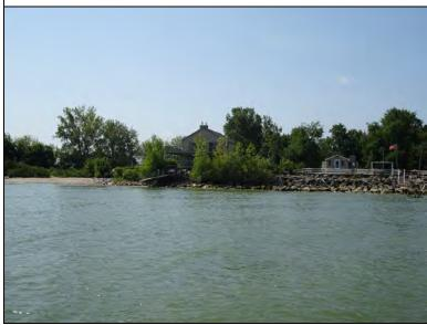
Inspect ID: OH29\_2020\_r\_0018 Title: USACE\_CELRB\_OH29\_2020\_r\_0018\_2.jpg Rated Item: 12. Riprap Revetments & Bank Protection Caption: Rating: Unacceptable; Remarks: Woody vegetation in riprap on levee waterside slope at 12763 Lagoon Drive, near Wards Canal.; Action: Remove woody vegetation from riprap. Perform regular maintenance to prevent further unwanted vegetation development.; Station\_1: -1+53; Station\_2: 0+10
