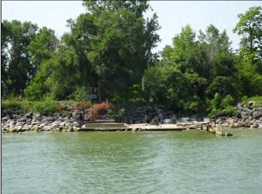
**Inspect ID:** OH29\_2020\_r\_0023 **Title:** USACE\_CELRB\_OH29\_2020\_r\_0023\_2.jpg **Rated Item:** 1. Unwanted Vegetation Growth **Caption:** Rating: Unacceptable; Remarks: Trees and woody vegetation on levee landside slope and crown at concrete slab, just west of 12153 Corduroy Road.; Action: Remove trees and woody vegetation. Perform regular maintenance to prevent further unwanted vegetation development.; Station\_1: 50+60
