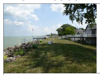
**Inspect ID:** OH29\_2020\_r\_0047 **Title:** USACE\_CELRB\_OH29\_2020\_r\_0047\_1.jpg **Rated Item:** 3. Encroachments **Caption:** Rating: Minimally Acceptable; Remarks: Unauthorized encroachments on both side slopes and crown of levee along multiple reaches of the project.; Action: Sponsor is coordinating with USACE to document and resolve encroachments.; Station\_1: 152+90
