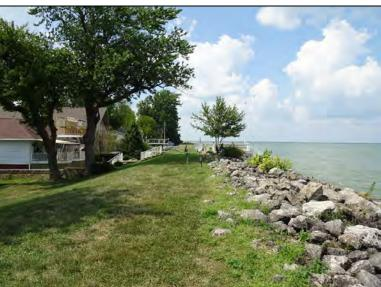
**Inspect ID:** OH29\_2020\_r\_0047 **Title:** USACE\_CELRB\_OH29\_2020\_r\_0047\_2.jpg **Rated Item:** 3. Encroachments **Caption:** Rating: Minimally Acceptable; Remarks: Unauthorized encroachments on both side slopes and crown of levee along multiple reaches of the project.; Action: Sponsor is coordinating with USACE to document and resolve encroachments.; Station\_1: 152+90
