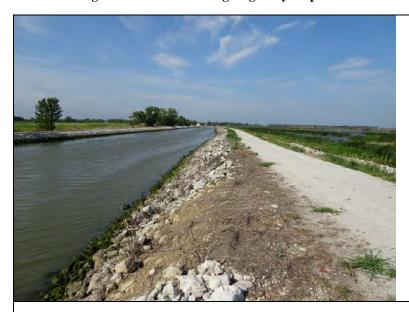
Inspect ID: OH29\_2020\_r\_0002 Title: USACE\_CELRB\_OH29\_2020\_r\_0002\_1.jpg Rated Item: 12. Riprap Revetments & Bank Protection Caption: Rating: Acceptable; Remarks: Riprap on levee waterside slope from Toulon Drive to project limit.; Action: NA; Station\_1: -47+80; Station\_2: -11+00
